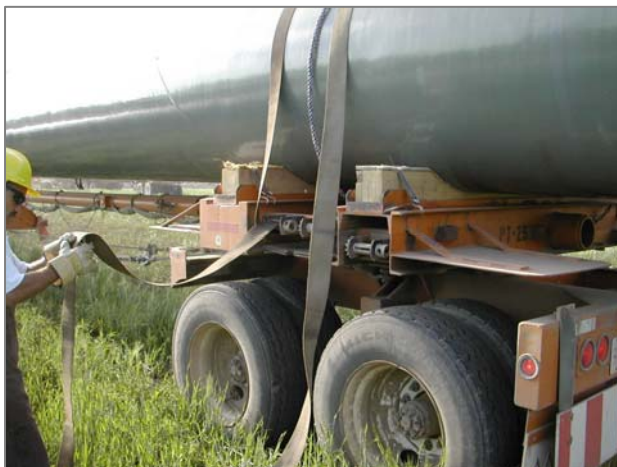
Photo courtesy of Premay Pipeline
